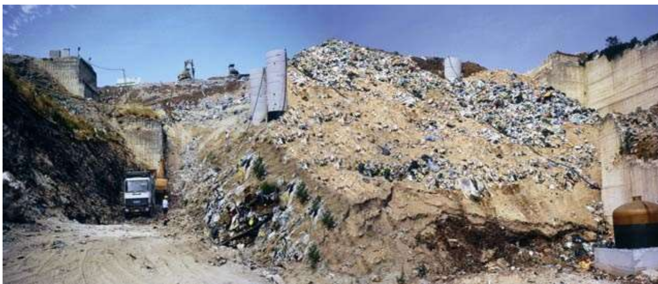
Consolidation by volumetric recovery of the South-East side of the "Pariti 2" landfill of Manfredonia (FG)- Overview of the initial state and final state
