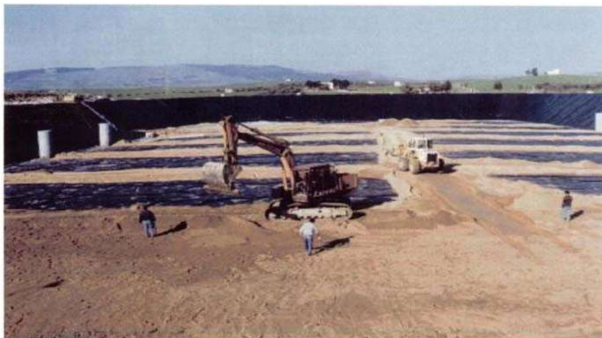
Waterproofing phase of the tank of the IV sector of the landfill
