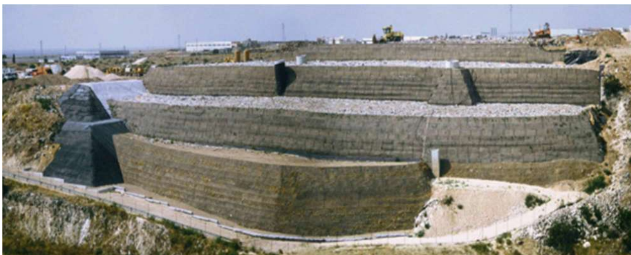
Consolidation by volumetric recovery of the South-East side of the "Pariti 2" landfill of Manfredonia (FG)- Overview of the initial state and final state
