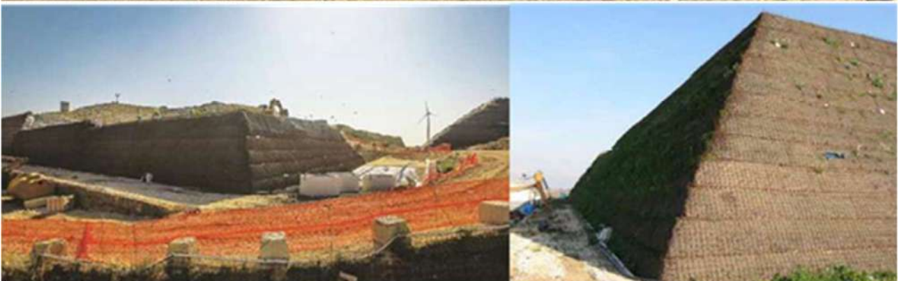
Overview of the construction of the containment structure and the viability in the "Passo Breccioso" landfill in Foggia
