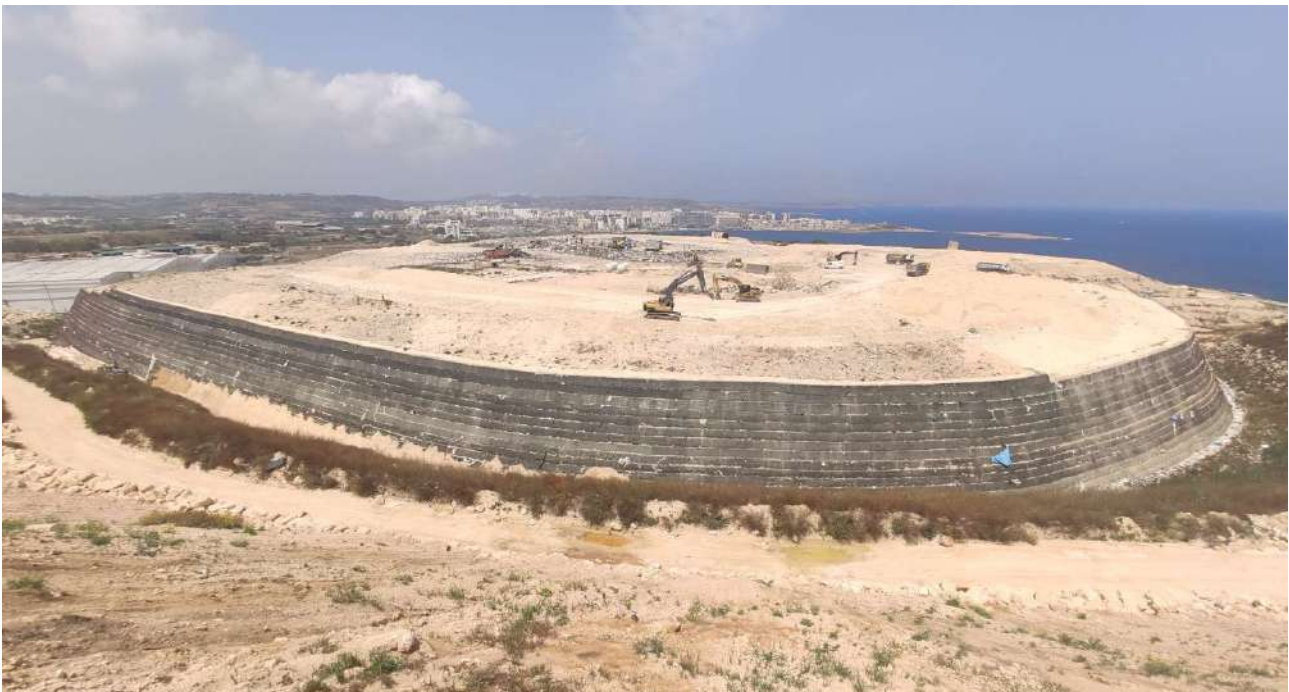
Detail of the recovery intervention in the Ghallis landfill, Ecohive Complex, Malta
