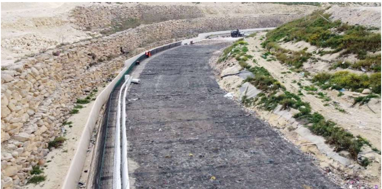
Formation of the containment structure of the Malta landfill - south/south - east side
